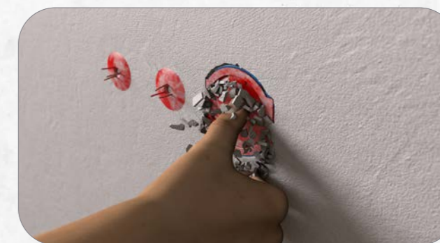
6. Signal Pins ensure quick location. Push the cover (P722) in with your finger or screwdriver. When it pops outwards, a clean contour is created without offsets in the plaster. Then remove the cover (P722).
