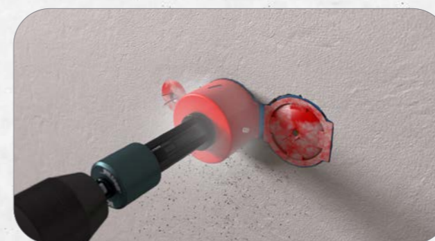
7. Alternatively, expose the Plaster Cover with a 68 mm Hole Saw (P797) and remove it.
