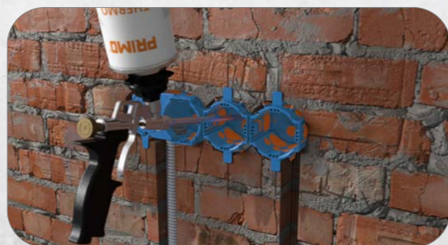
4. Use the Foam Pistol (P719) to break out the predetermined breaking point in the rear of the box and inject the foam (P717) until the box is completely enclosed. After 30 minutes, the foam is cut-resistant.
