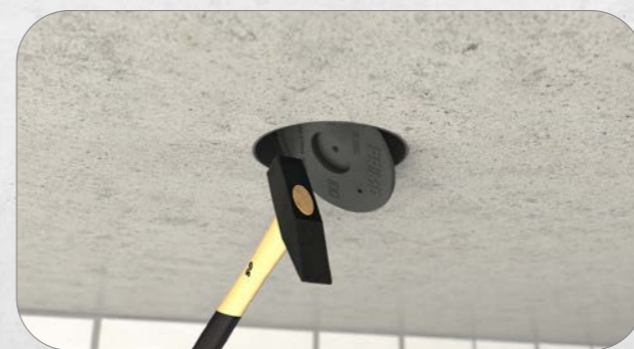
5. Open the Front Part with a hammer blow after concreting.
