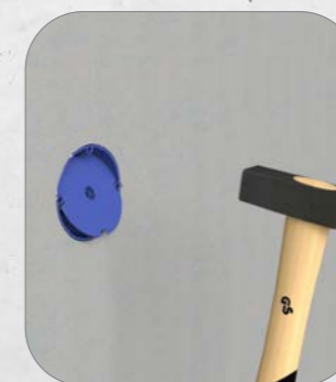
11. Break out the cover with a hammer.
