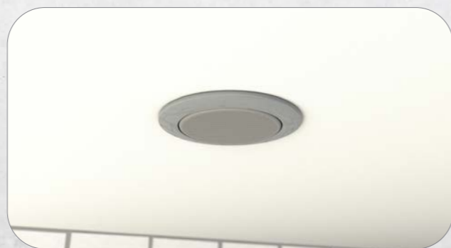
12. Install any built-in devices such as luminaires or loudspeakers.
