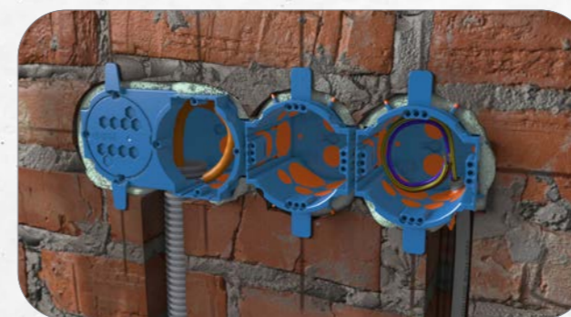
5. Pierce the Cable-Plopp with the cable and thus insert the cable entirely without tools.
