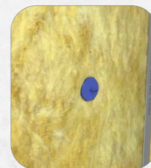
5. Attach insulation wool.
