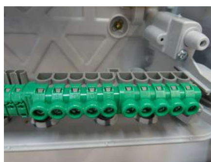
Earth terminal block: screw terminals
