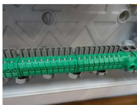
Earth terminal block: automatic connection
